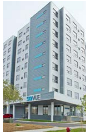
SkyVue 3,890 SF for Lease in Mixed-Use Project
